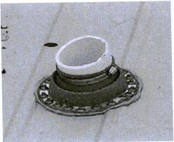
2. Add coupling and extend height of plumbing vent – 1 location.
